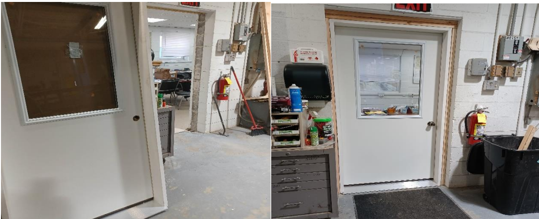
SHOP DOOR REPLACED
