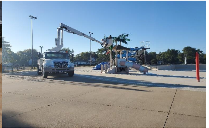
VANDALISM DEPOT PARK
