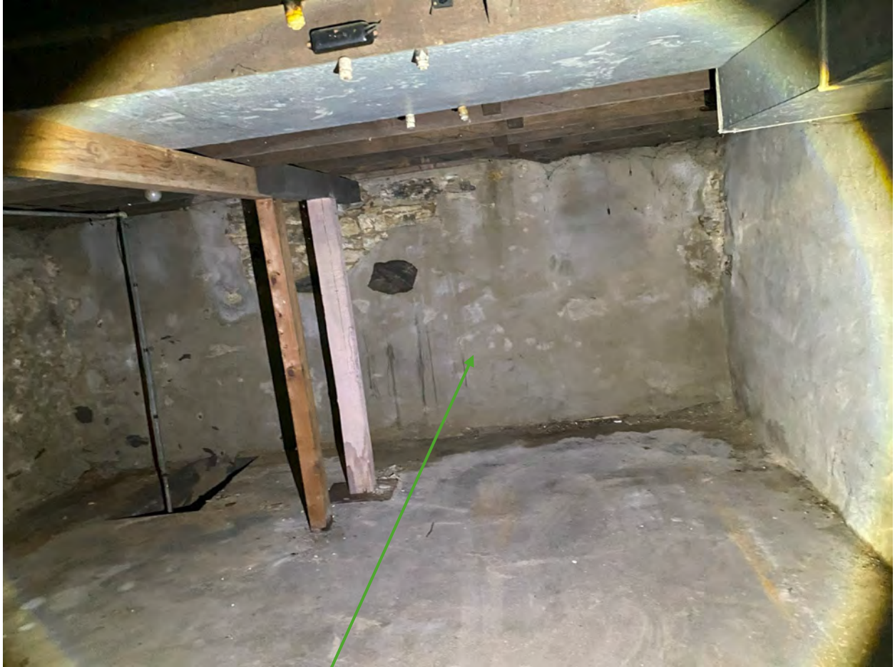
West foundation wall
