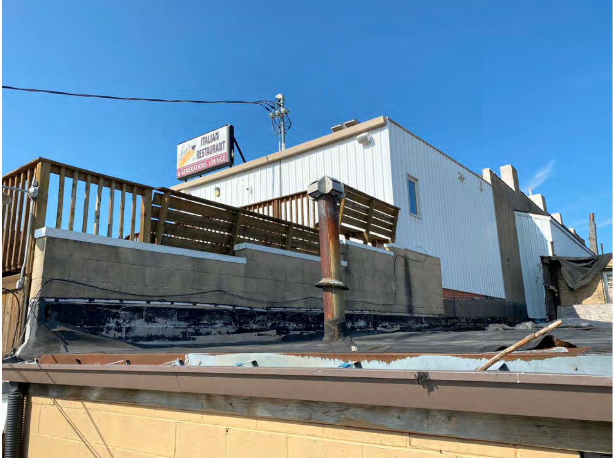
Southeast wall/parapet-wall showing deck buildout
