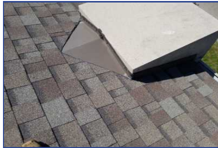
Section A - Deficiency #2 Improperly flashed pillars
