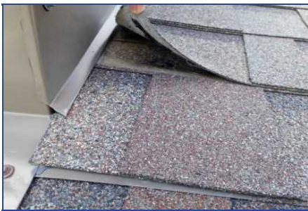
Section B - Deficiency #5 Poorly installed flashing
