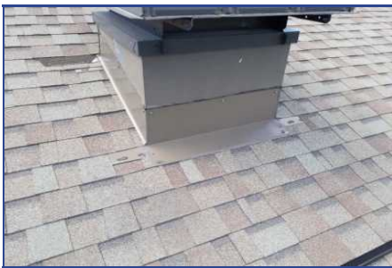
Section B - Deficiency #5 Poorly installed flashing
