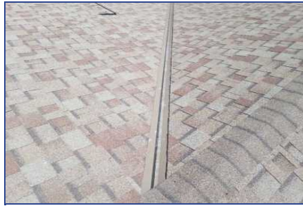
Section B - Deficiency #3 Deteriorated valley tin
