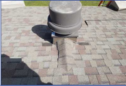
Section B - Deficiency #6 Curb improperly slashed
