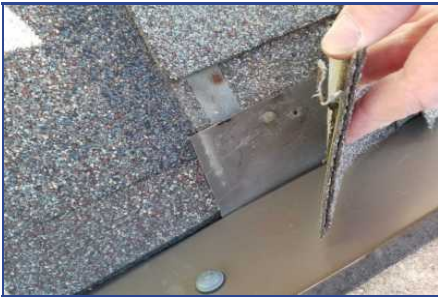
Section A - Deficiency #2 Improperly flashed pillars
