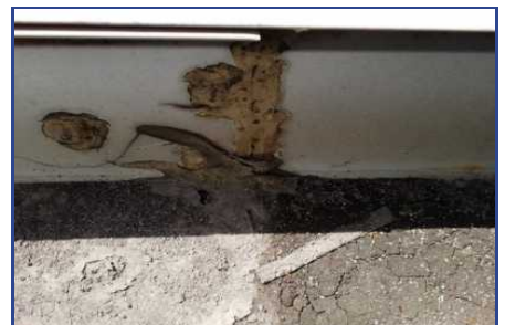
Section B - Deficiency #2 Metal flashing sealant deteriorated or missing
