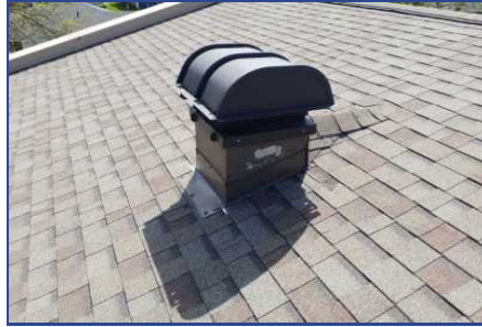
Section B - Deficiency #6 Curb improperly slashed
