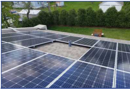
Section B - Deficiency #4 Improper Plumbing pipe flashing
