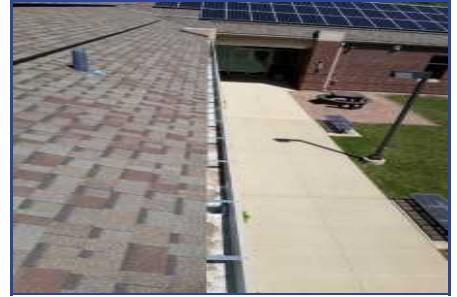
Section A - Deficiency #6 Failing sealant
