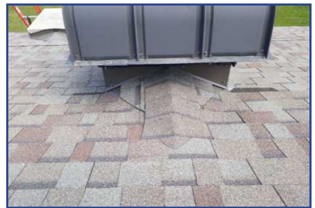
Section B - Deficiency #5 Poorly installed flashing
