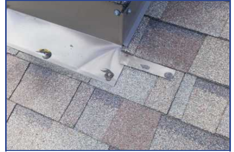
Section B - Deficiency #6 Curb improperly slashed
