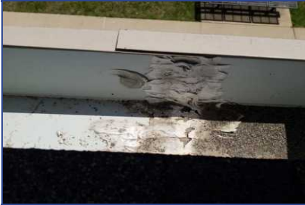
Section A - Deficiency #6 Failing sealant
