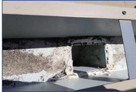
Section A - Deficiency #6 Failing sealant
