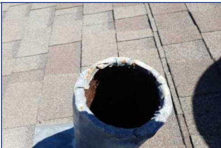
Section B - Deficiency #1 Rusted Lead Top
