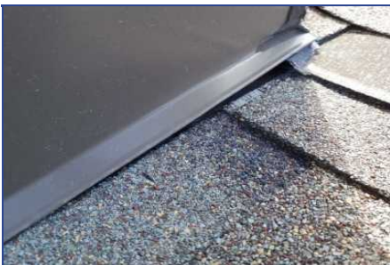
Section B - Deficiency #6 Curb improperly slashed
