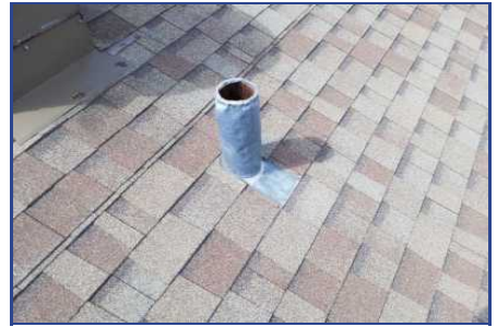
Section B - Deficiency #4 Improper Plumbing pipe flashing
