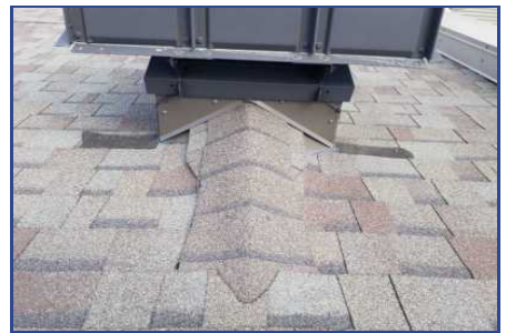
Section B - Deficiency #5 Poorly installed flashing
