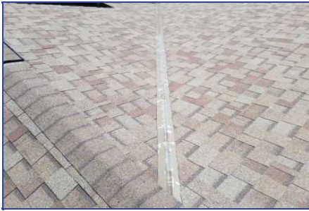
Section B - Deficiency #3 Deteriorated valley tin
