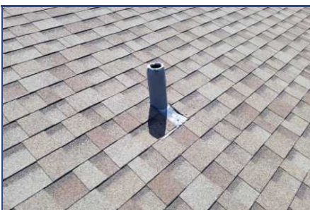
Section A - Deficiency #4 Improper flashing on Plumbing stack
