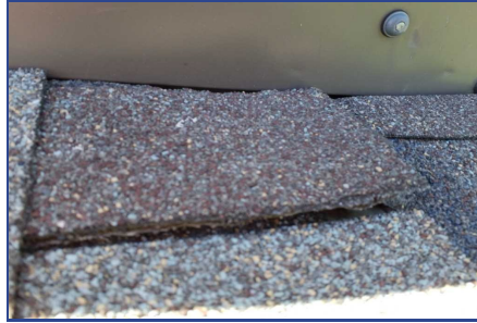
Section A - Deficiency #2 Improperly flashed pillars
