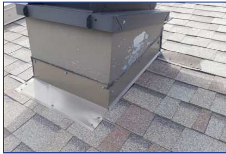
Section B - Deficiency #5 Poorly installed flashing
