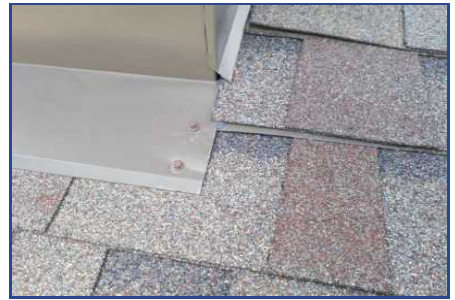
Section B - Deficiency #5 Poorly installed flashing
