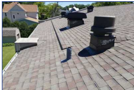
Section B - Deficiency #1 Rusted Lead Top
