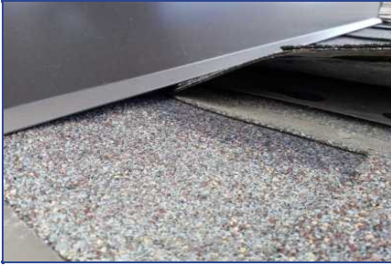
Section B - Deficiency #5 Poorly installed flashing
