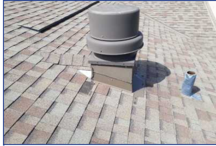
Section B - Deficiency #6 Curb improperly slashed
