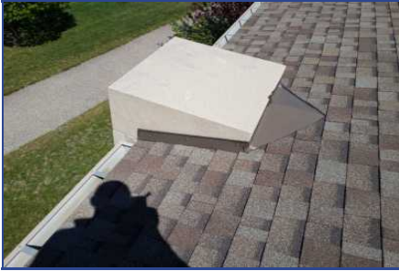
Section A - Deficiency #2 Improperly flashed pillars
