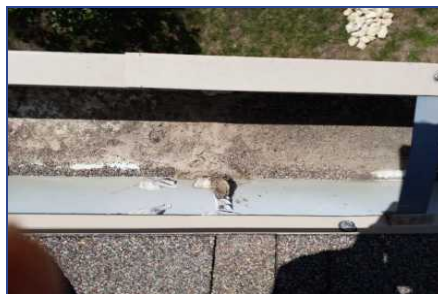
Section B - Deficiency #2 Metal flashing sealant deteriorated or missing
