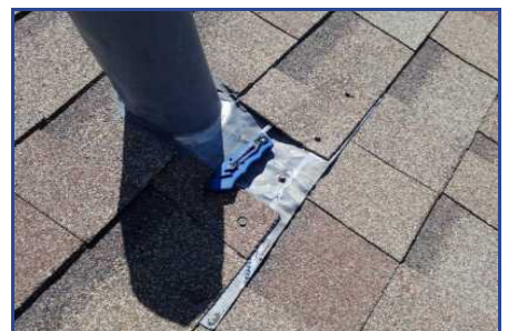
Section A - Deficiency #4 Improper flashing on Plumbing stack
