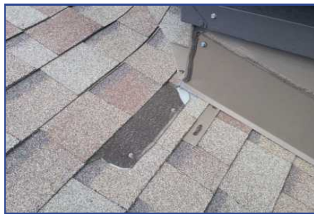
Section B - Deficiency #5 Poorly installed flashing
