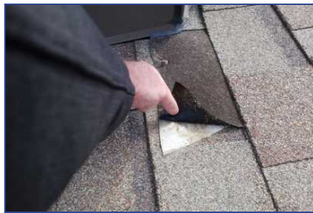
Section B - Deficiency #5 Poorly installed flashing
