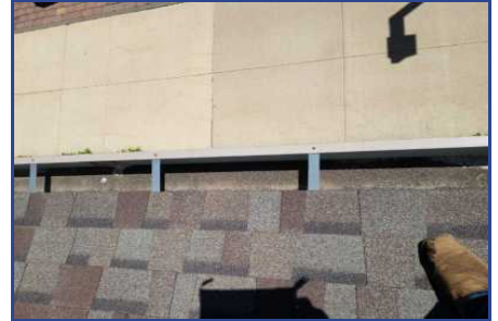
Section A - Deficiency #6 Failing sealant
