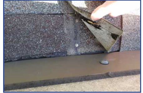
Section A - Deficiency #2 Improperly flashed pillars
