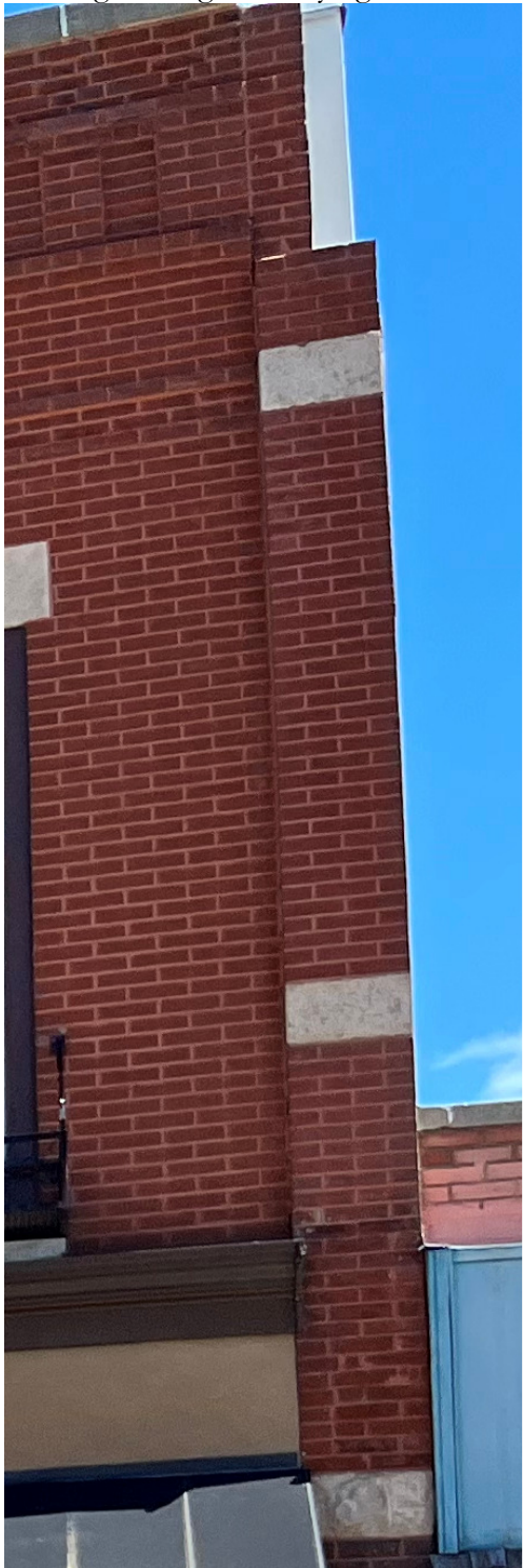
Figure 1: Joint prior to demolition
