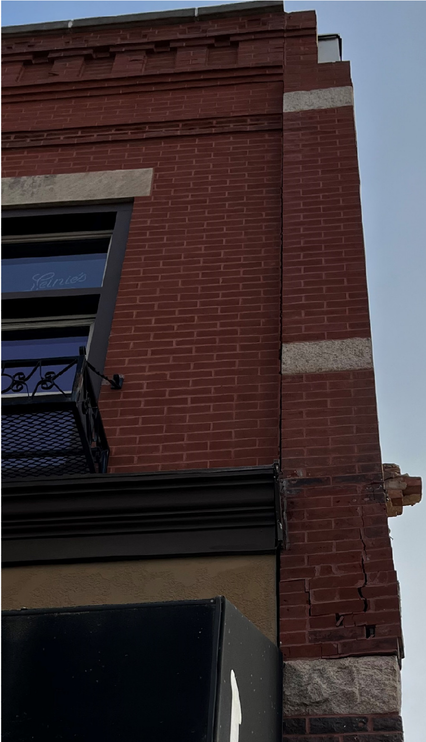
Figure 2: Opening in joint after demolition
