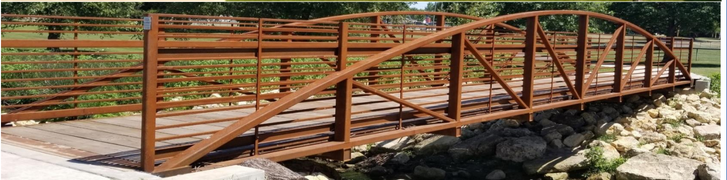
Segment 1 – Great Western Avenue Area NW
