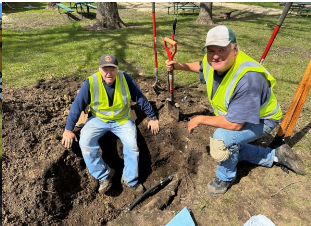
WATER LINE FIX
