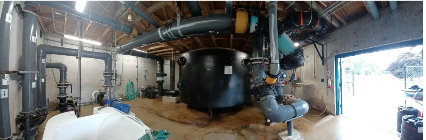
FILTER/PIPING REMOVAL COMPLETED
