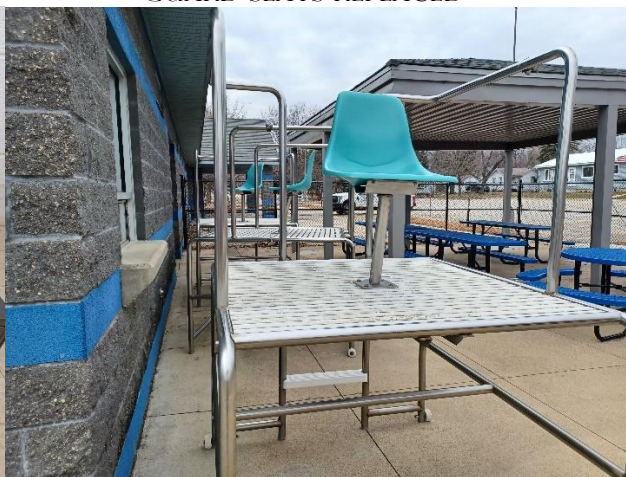
GUARD SEATS REPLACED
