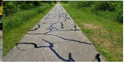
Crack sealing east trail
