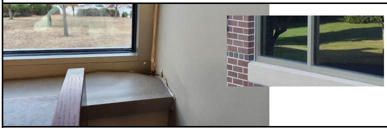
Project Description: Repair window leaks and window sills by removing the existing windows and replacing the sills. The glass and storefront framing will be re-used.
