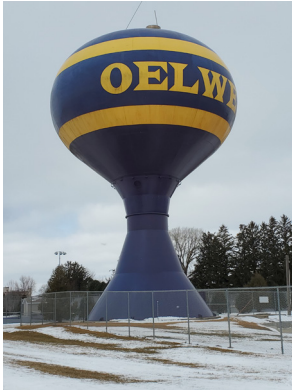
Oelwein Water Tower
