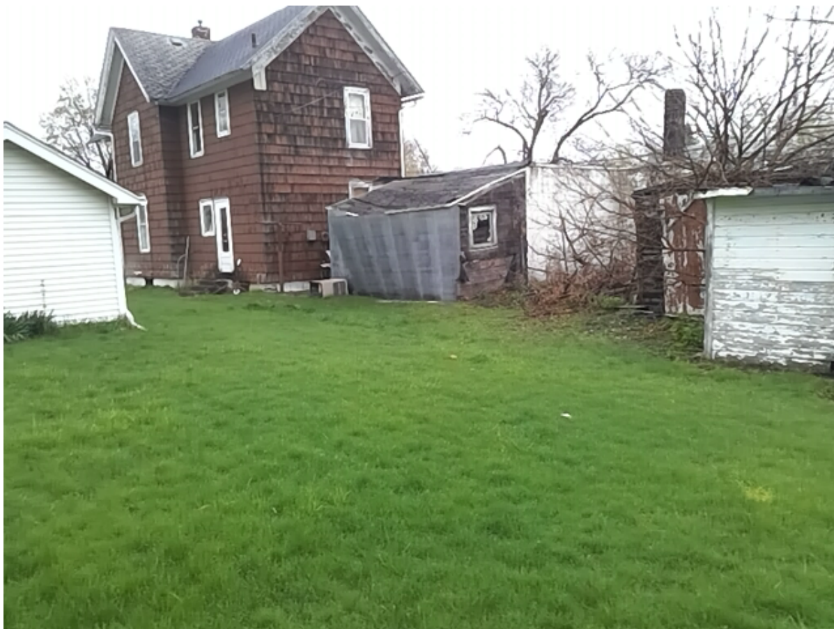
Photo: Collapsed structure
