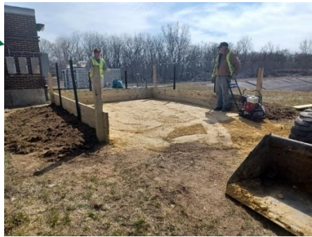
GRAVEL BED CONSTRUCTION COMPLETED
