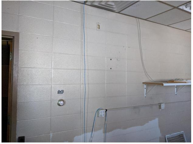
The second window would be another service window. This wall is a non-load bearing sheet rock stud wall. Same dimensions as the window above.
