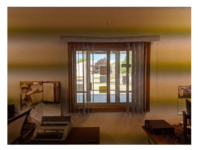
The last option would be for a new main service window. It would match the other service windows and be removing an older window. This wall is non-load bearing block. Same size as the other service windows.
