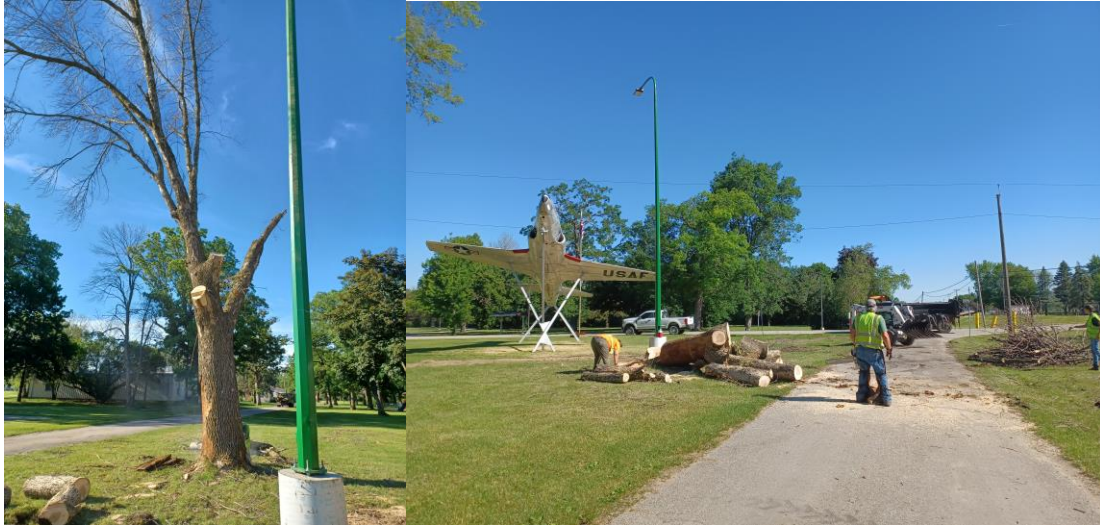
ASH TREE REMOVAL - WINGS
