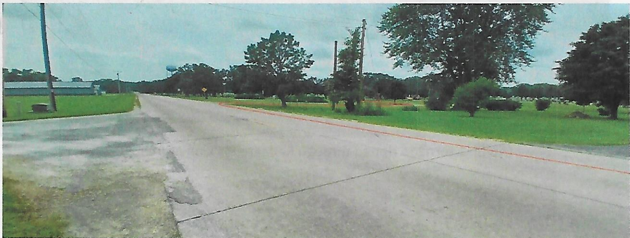
13 th Avenue NW and 2 nd Street NW
