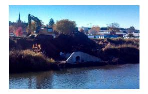
Repair plans and methods needed to accommodate the possibility of flooding occurring during construction activities. MSA required the contractor to close the gap in the levee any time crews were not on site and incorporate suitable temporary erosion control practices to protect the waterward side of the levee, should flooding occur while the levee was temporarily closed.
