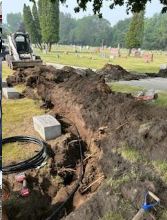
WATER LINE REPAIR
