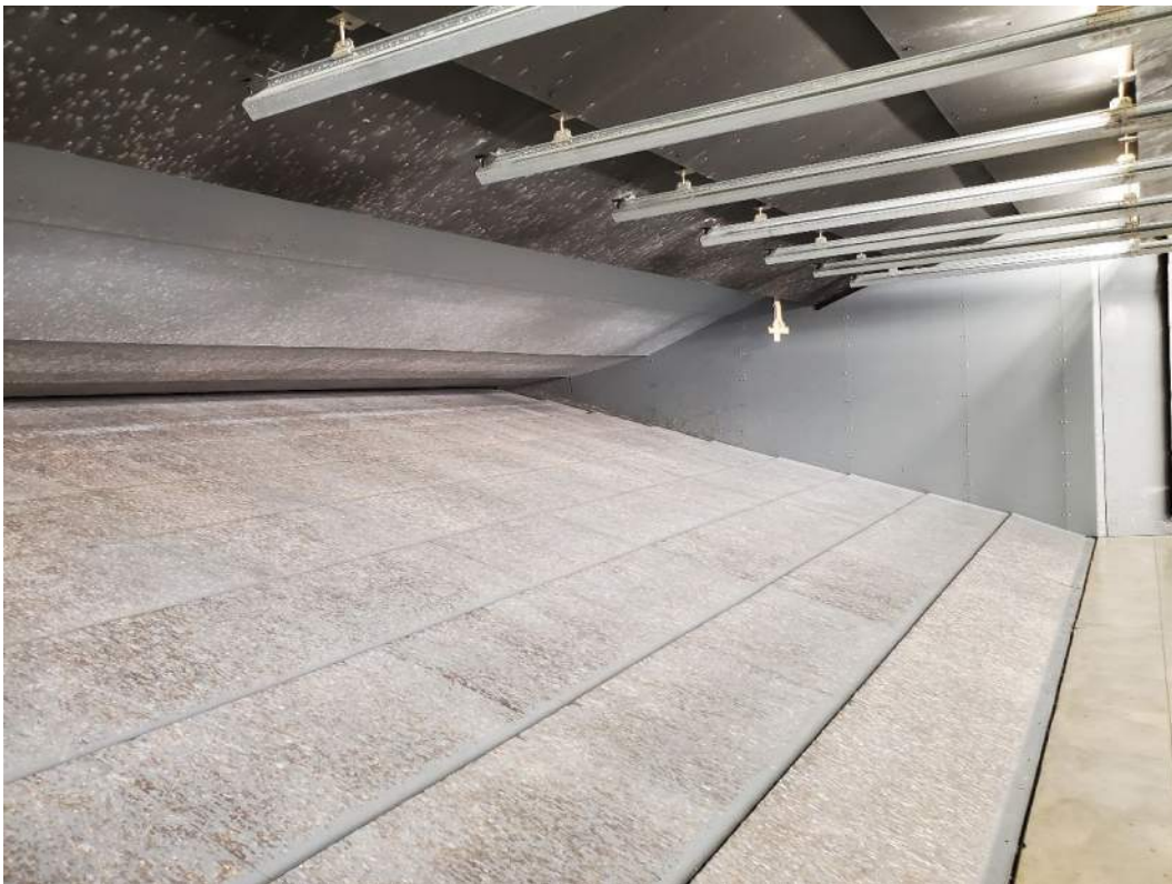
Photograph 19: Hero Center ammunition collection baffles
