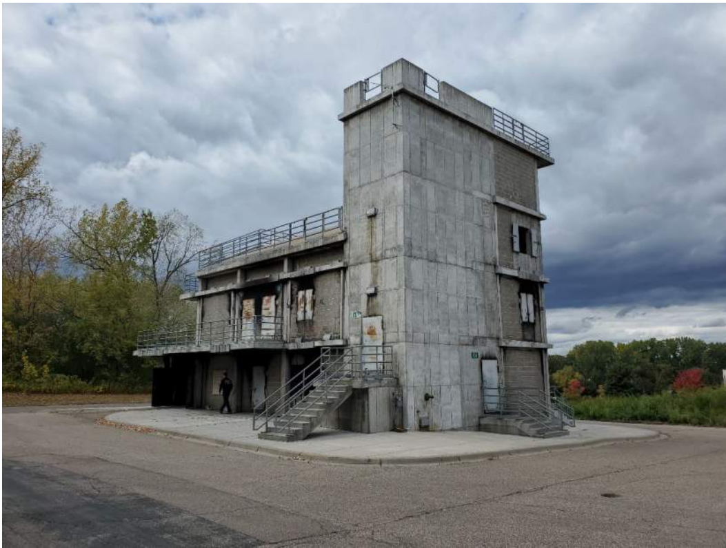
Photograph 24: South Metro tactical fire training tower
