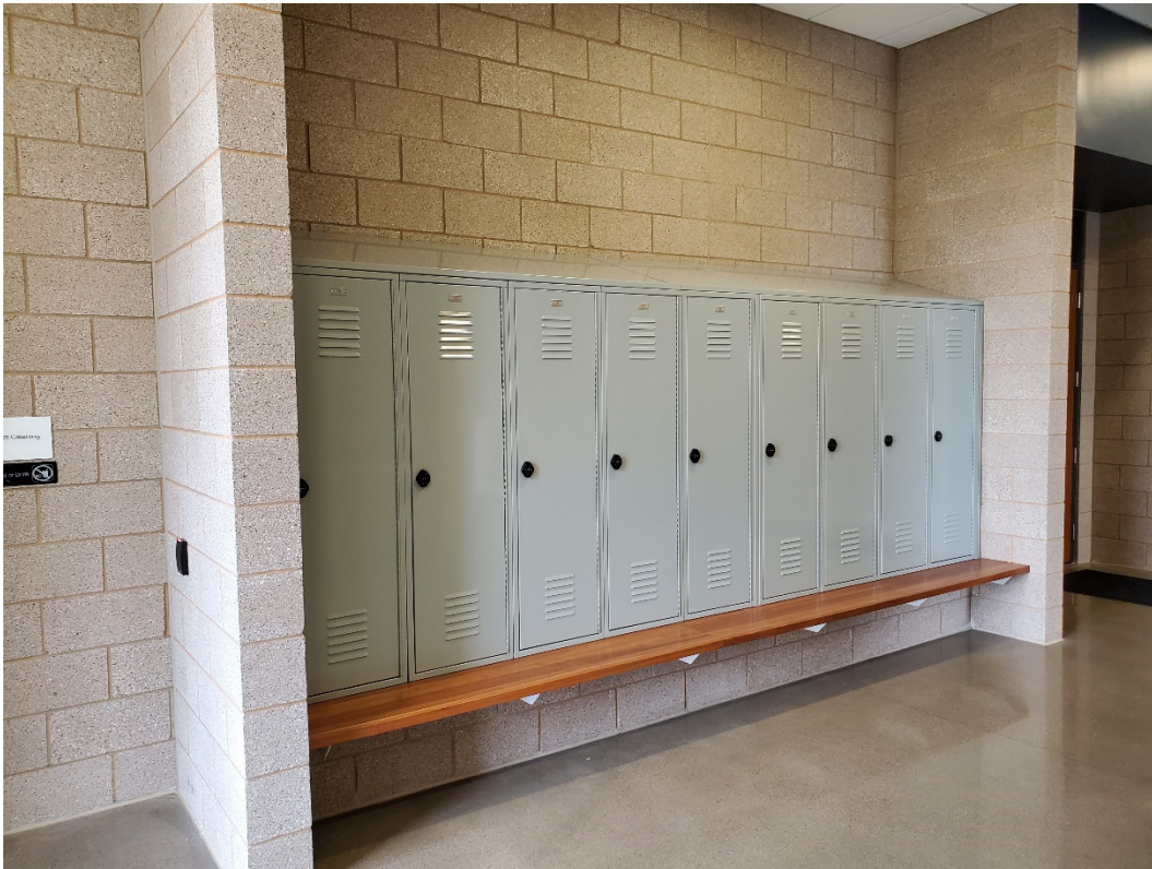
Photograph 21: Hero Center hall storage
