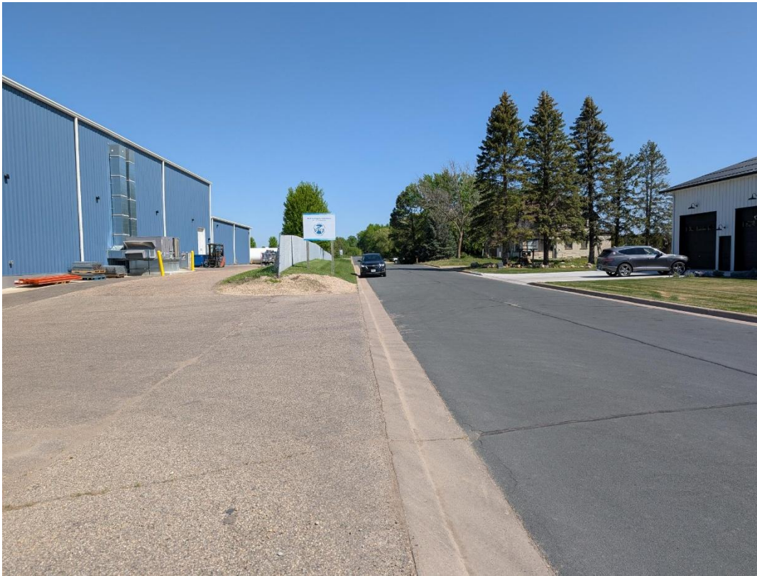
Looking north along 1 st Ave. NW – Temporary Gravel widened the approach to see if trucks could better make the turn.
