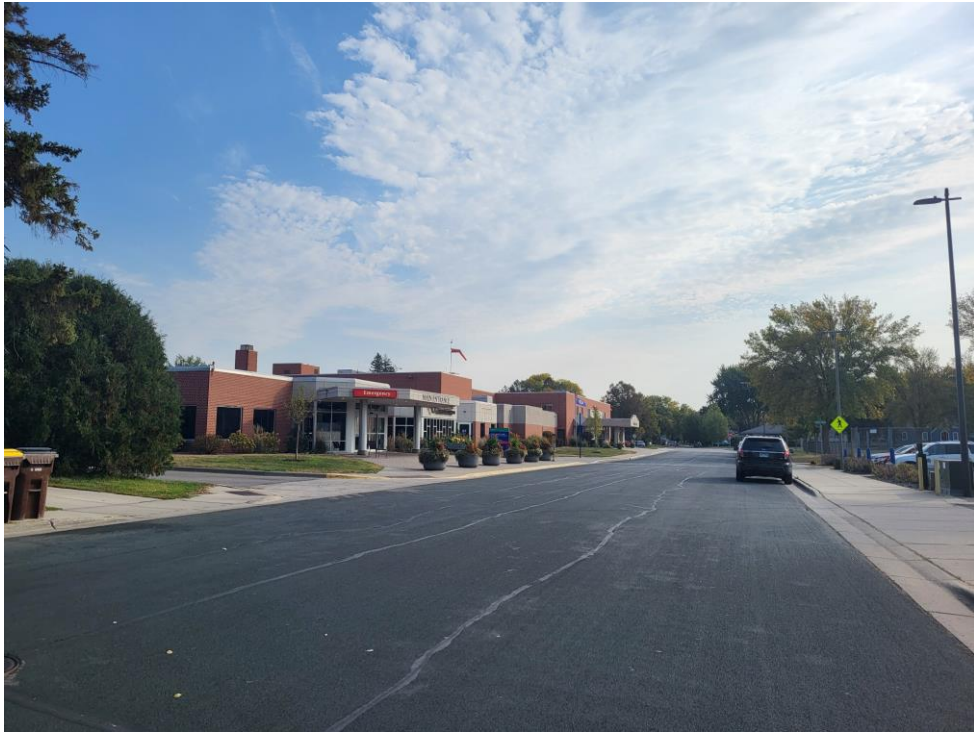
Looking NE from 2 nd Street NE at main entrances (patient parking lot on south side of 2 nd Street NE).
