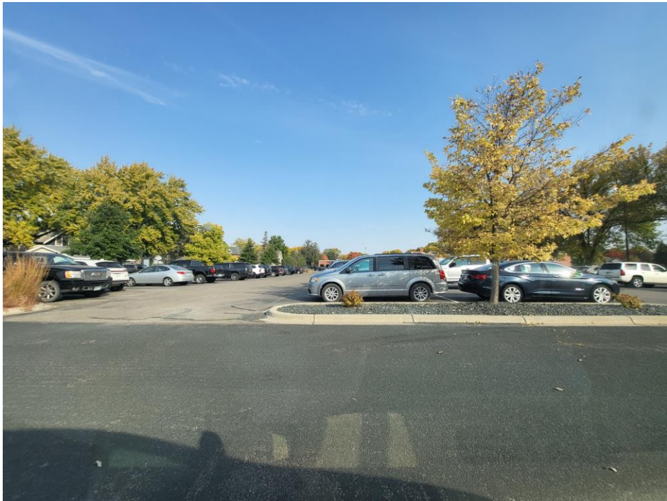
Looking North from the south edge of the 100 space patient parking lot.
