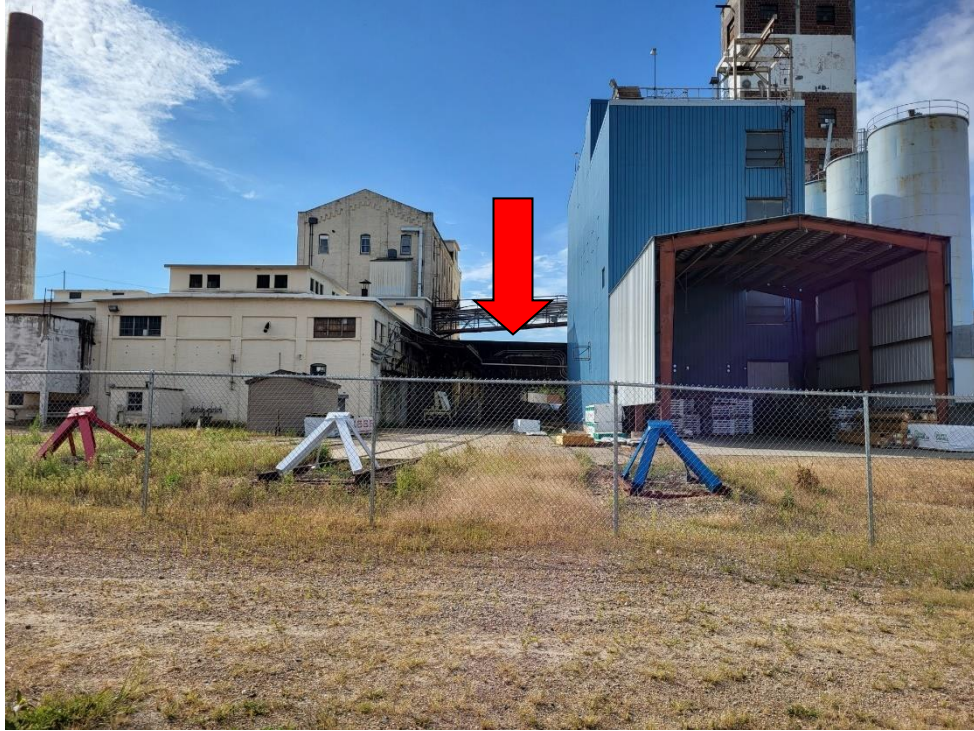
View of Canopy Area from Main St. W. (middle of the photo) – Other stored items in this photo must be moved to storage area under canopy.
