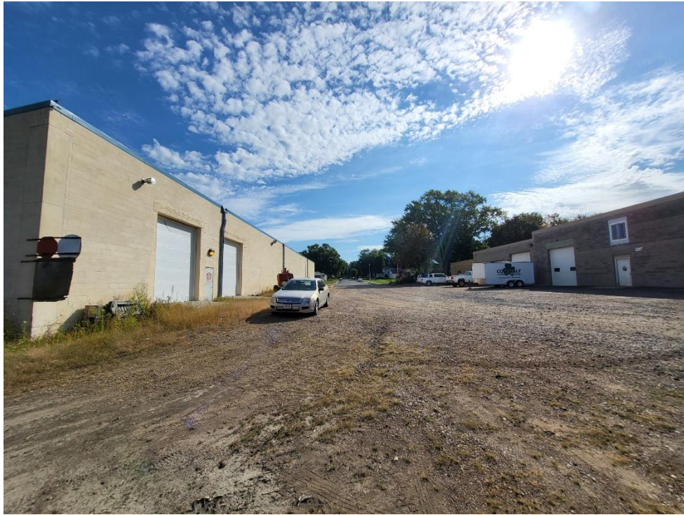
Looking east along 2 nd Street SW ROW from railroad spur.
