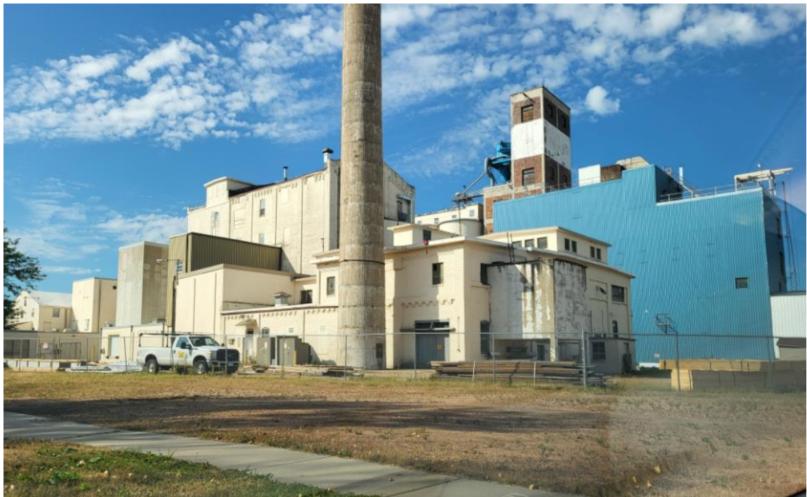
Looking at site from 2 nd Ave. SW (these exterior storage items must be removed and fence revised to only enclose storage or other areas not yet being rented/occupied).
