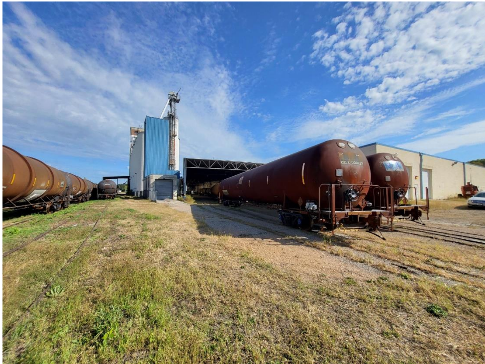
Looking north along Railroad spur towards south side of canopy storage area.
