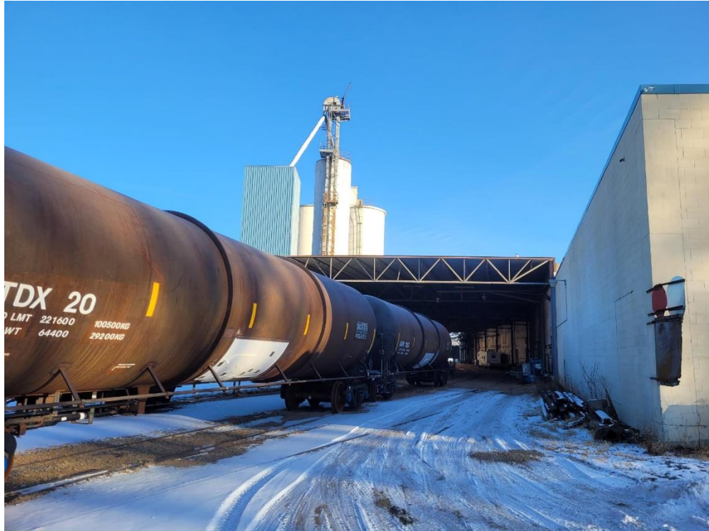
Looking North on the Rail Spur Towards the Southside of the Canopy Storage Area
