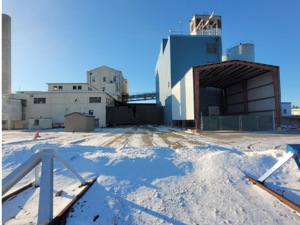
View of Canopy Area from Main St W – Sound Blanket Currently Covering Front Entrance
