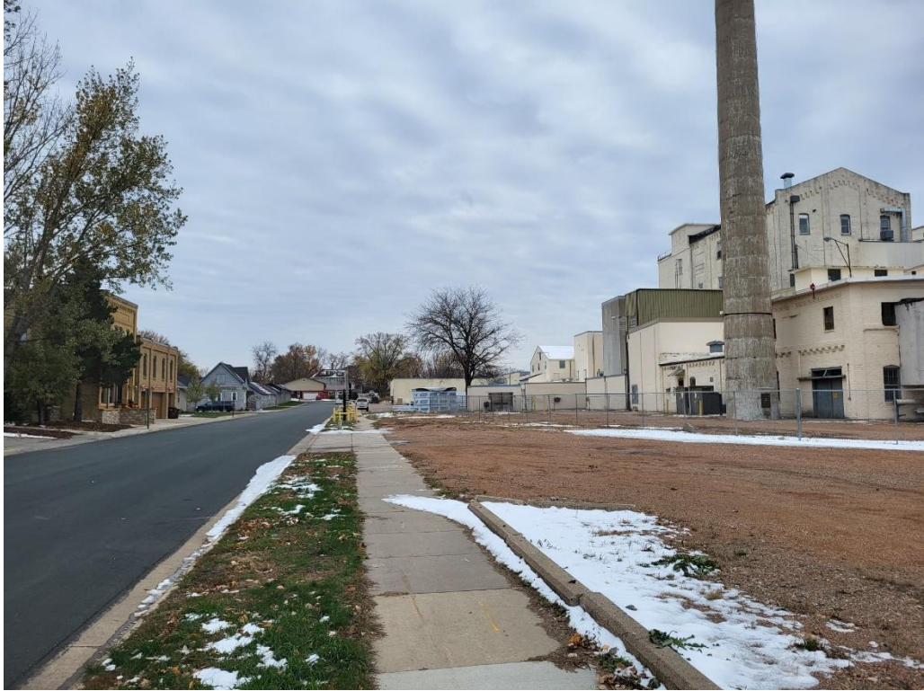
Looking south along 2 nd Ave. SW.
