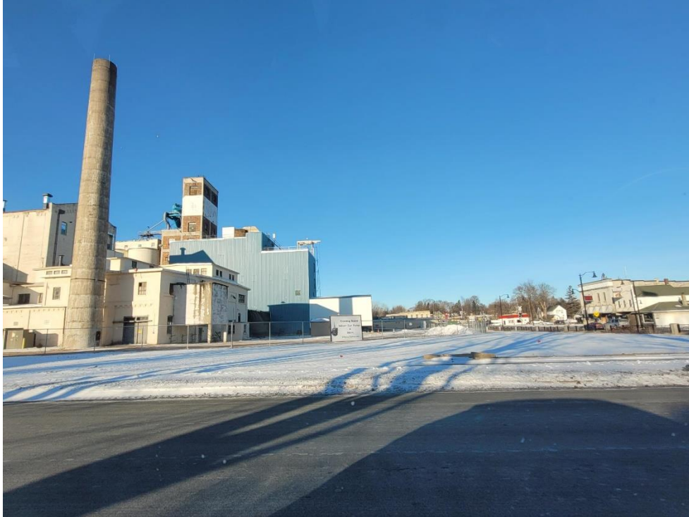
Looking West from 2 nd Ave SW
