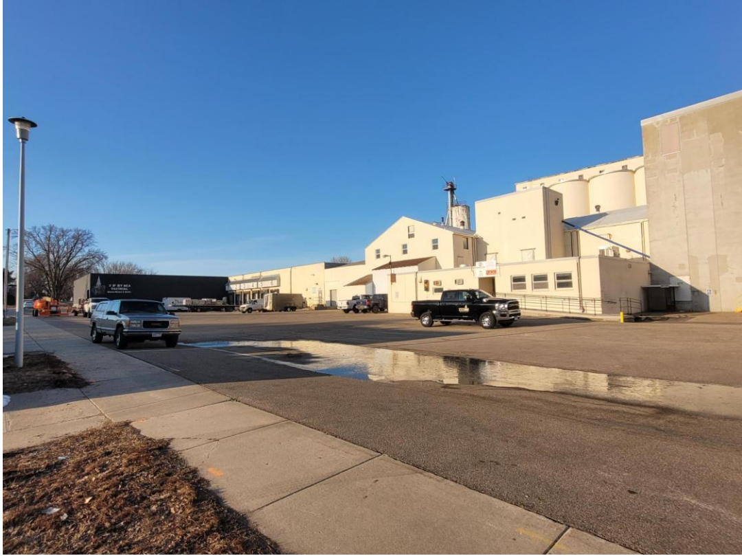
Picture of the Mill Looking West from 2 nd Ave SW
