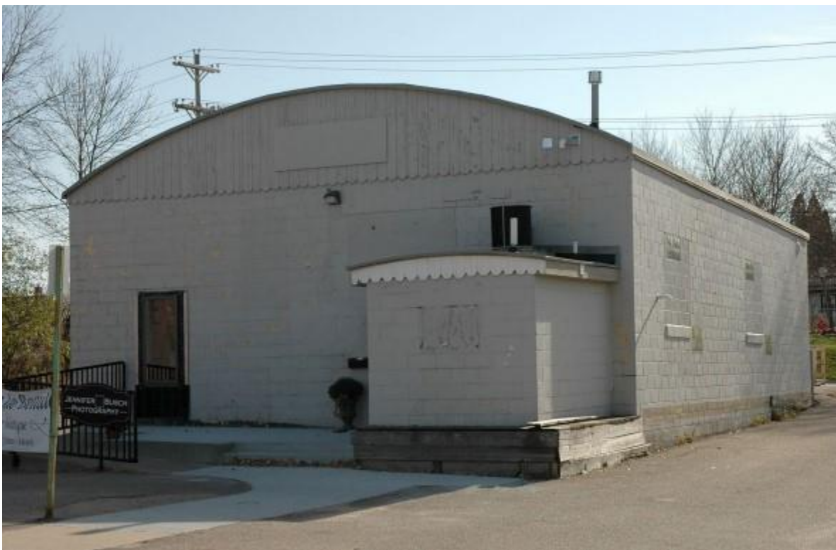
126 Main St W - Cement Block Cladding
