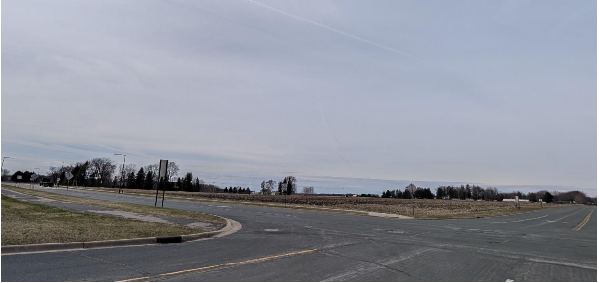
Looking SW from intersection of 1 st Street NW and 11 th Ave. NW
