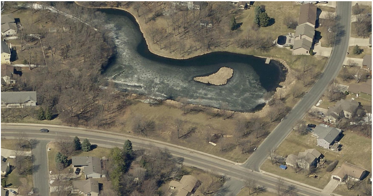
Oblique Air Photo – Looking North at the Property
