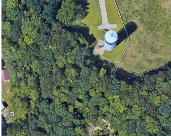
Figure 29. Jordan Water Tower and Eroding Bluff (imagery from 2019)
