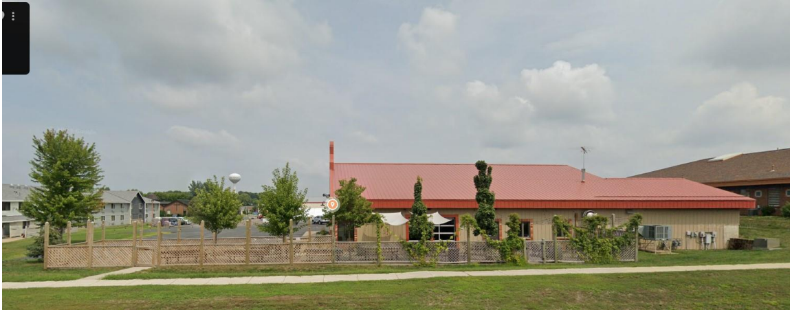
Giesenbrau Bier Co. Patio - Looking North from TH19/Main St – Google Street View
