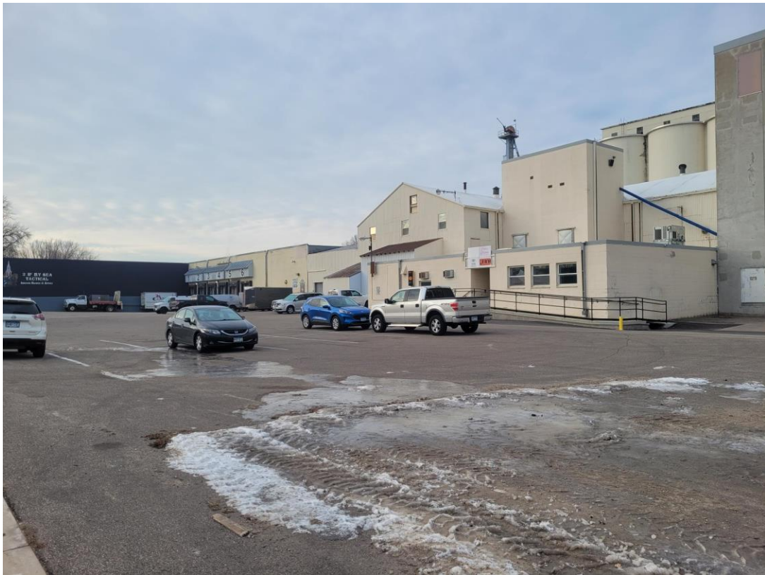
Looking Southwest Towards the Office Entrance and Accessible Ramp
