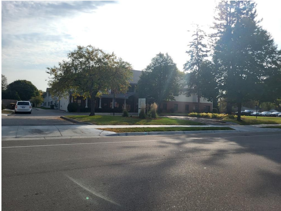
Looking at the east side of Columbus Ave. N. at Queens Court building which is across the street from the proposed addition.
