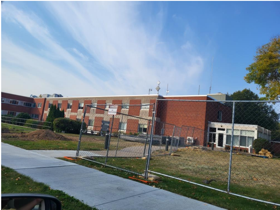
Looking SW from Columbus Ave. N. at the location of the proposed building addition.
