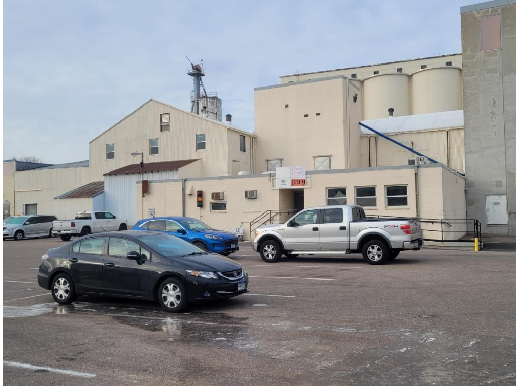
Looking West Towards the Office Entrance
