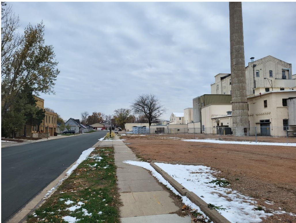
Looking south along 2 nd Ave. SW.
