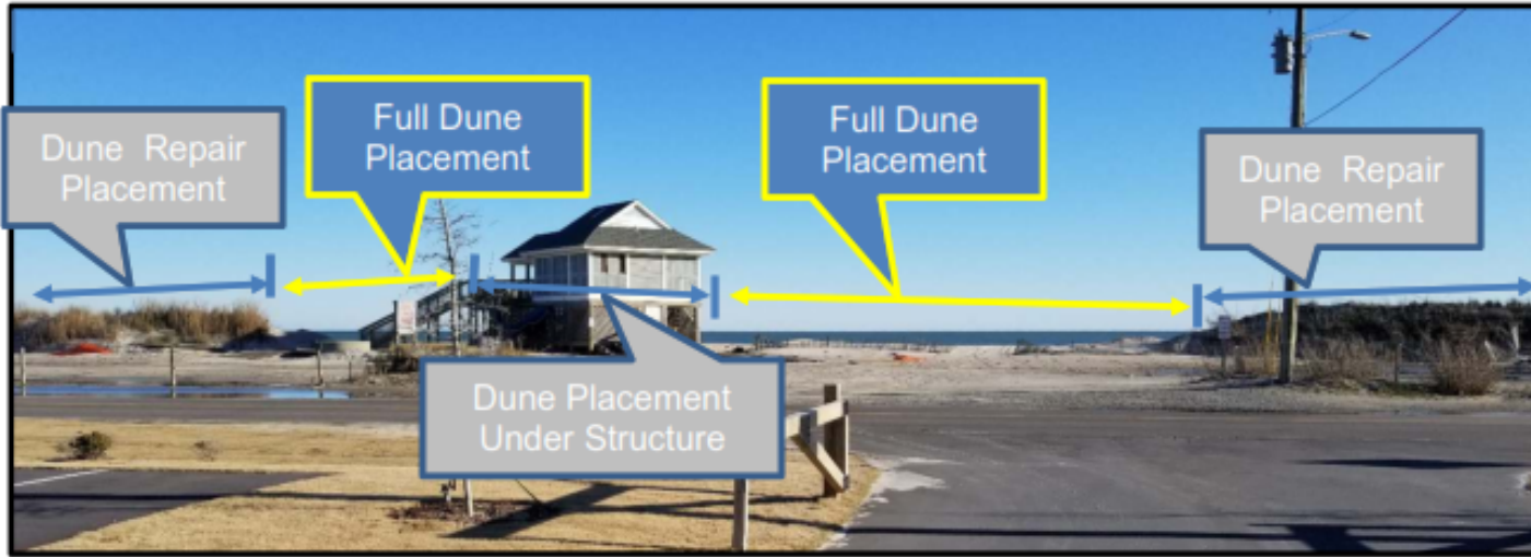
Figure 1: Dune Material Placement (photo taken February 3, 2021).
