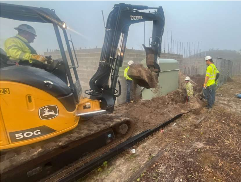
Here you can see the grading and silt fence repair required after they were finished
