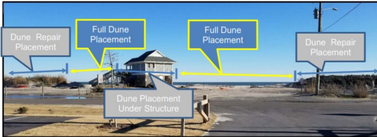
Figure 1: Dune Material Placement (photo taken February 3, 2021).
