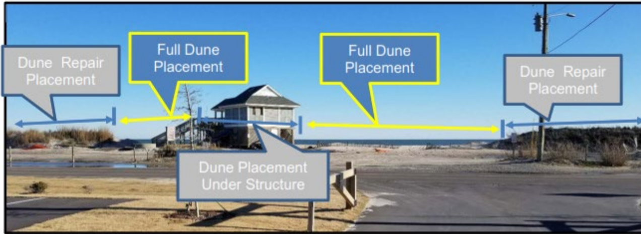
Figure 1: Dune Material Placement (photo taken February 3, 2021).
