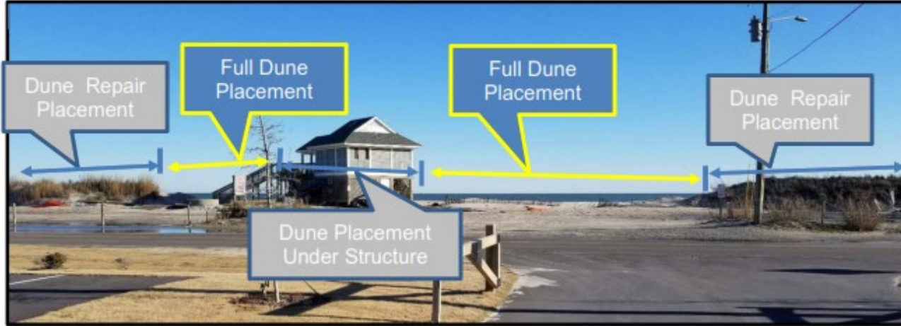
Figure 1: Dune Material Placement (photo taken February 3, 2021).
