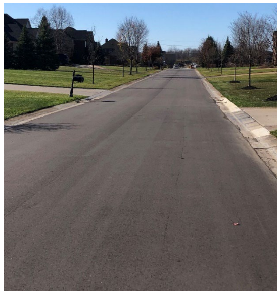
Park Place Drive - After
