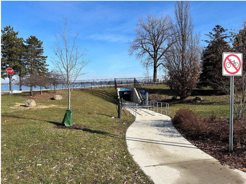
After – Park side (south)
