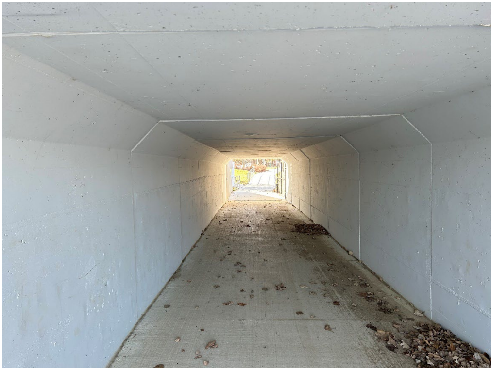
After – Inside tunnel
