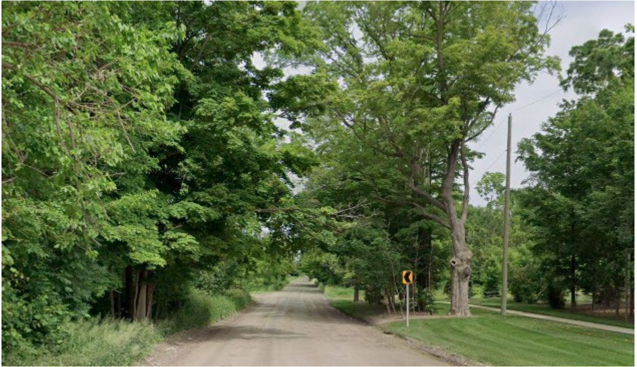
Before – 12 Mile east of Medina looking east.
