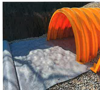
Looking down the Isolator Row Plus from the manhole opening, ADS Plus Fabric is shown between the chamber and stone base.
