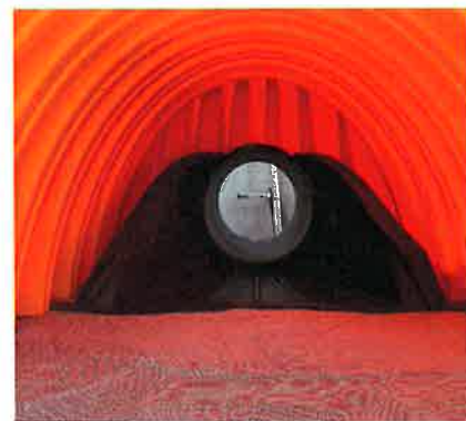
Looking down the Isolator Row Plus from the manhole opening, ADS Plus Fabric is shown between the chamber and stone base.
