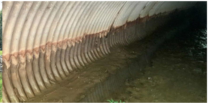
INTERIOR PIPE CONDITION Inspection photograph, June 2022
