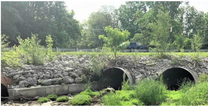
EXISTING FOUR-BARREL CROSSING Inspection photograph, June 2022
