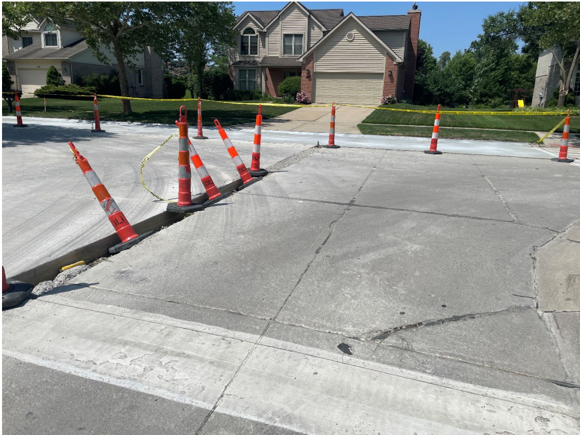
Before – Moorgate Street at Havergale Street
