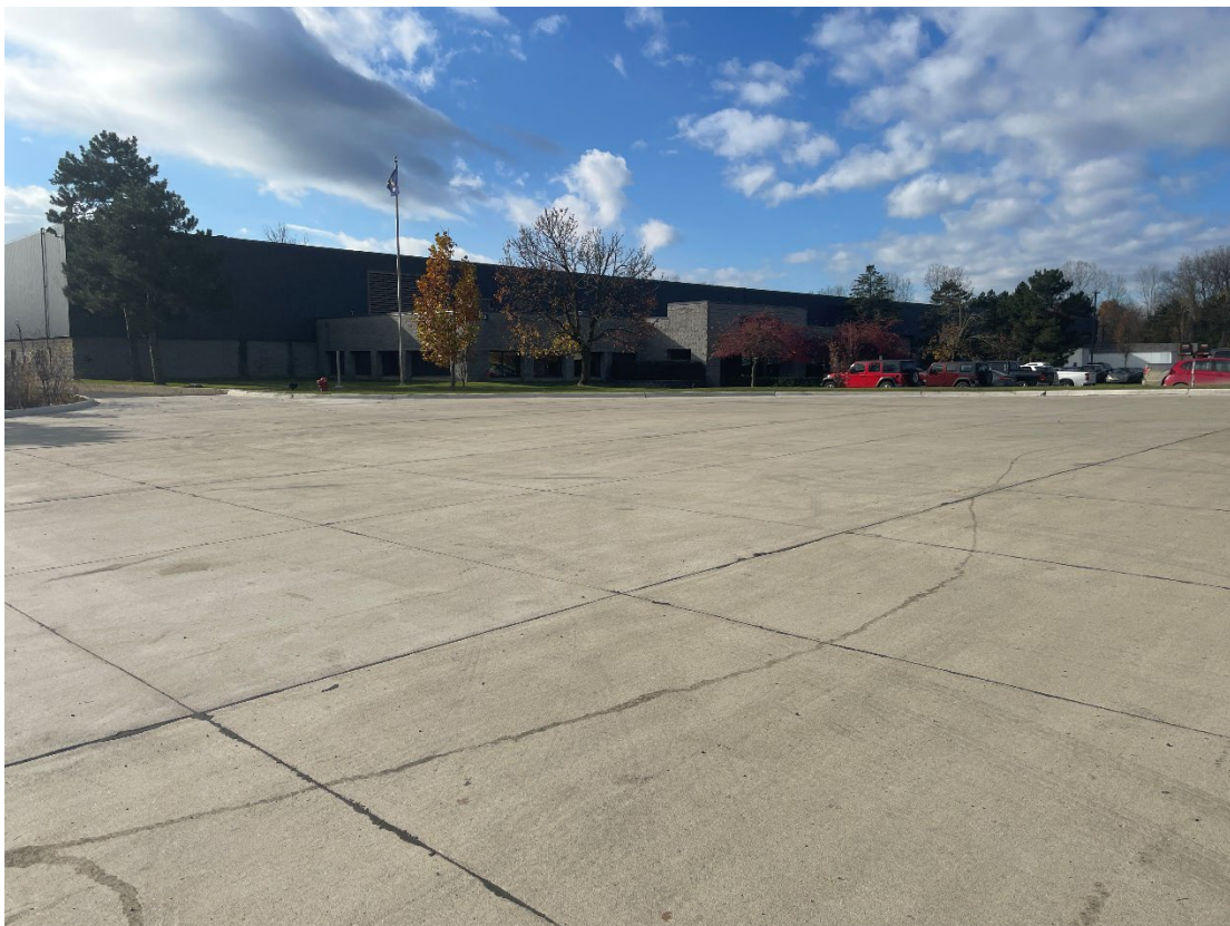
After – Gen-Mar Drive at cul-de-sac
