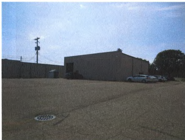
Property to the west
