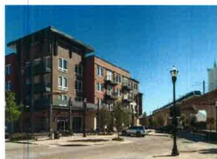
Multi-unit dwellings with first floor retail
