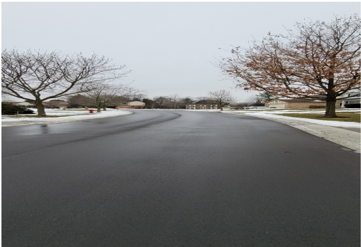
Orchard Ridge Subdivision – Hickory Grove - Completed
