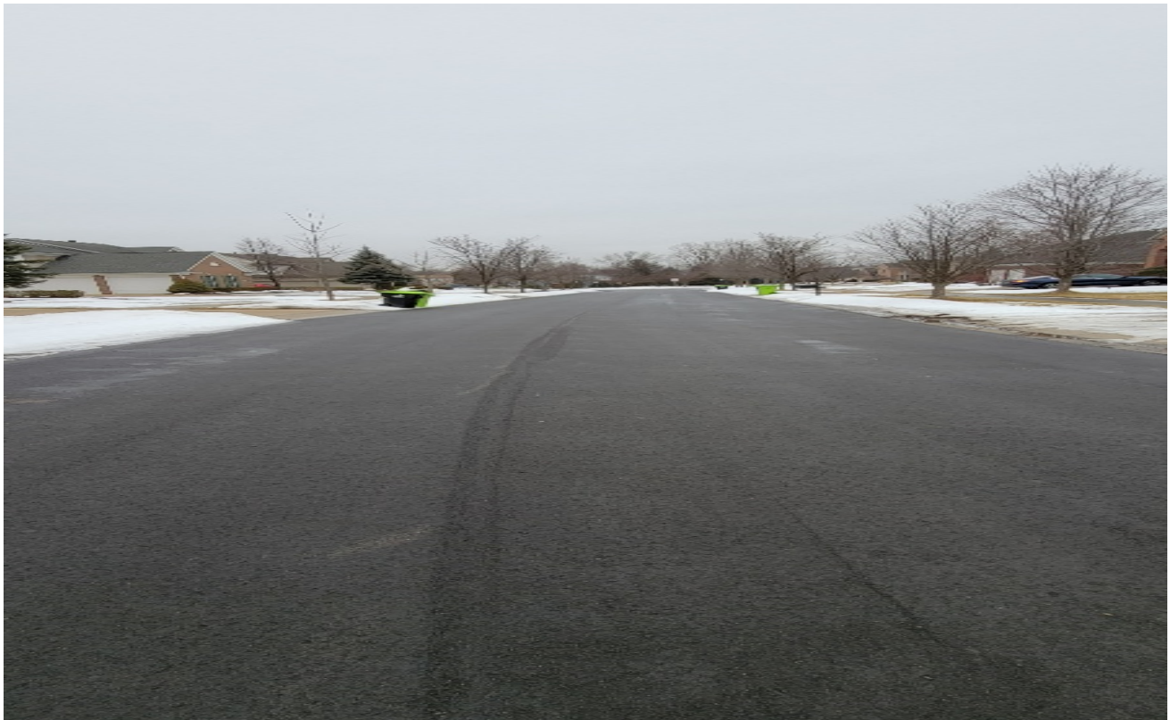
Brookhaven Subdivision – Myrtle Court off 10 Mile – Completed
