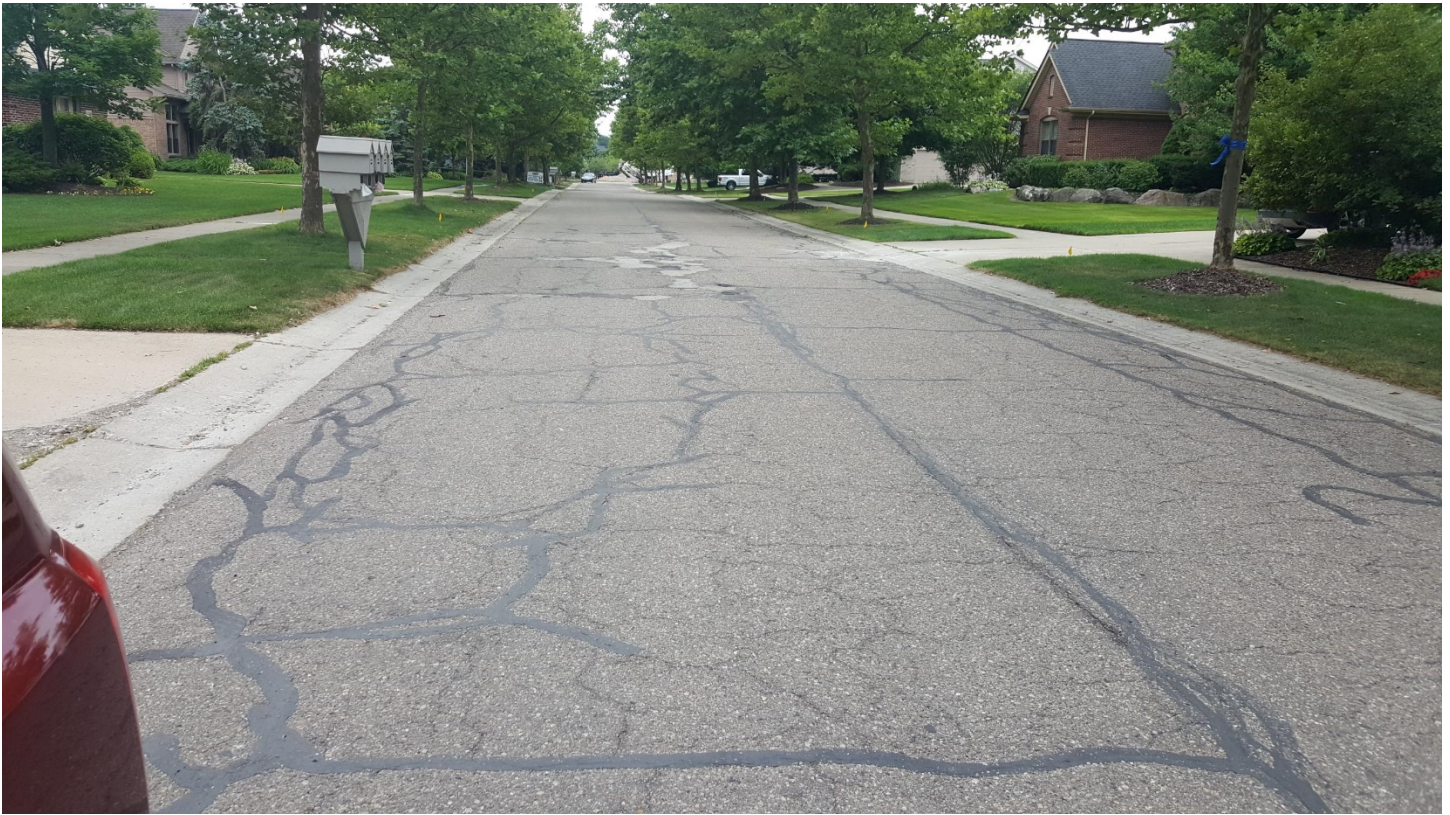
Greenwood Oaks Sub – Greenwich Drive – Pre-Construction
