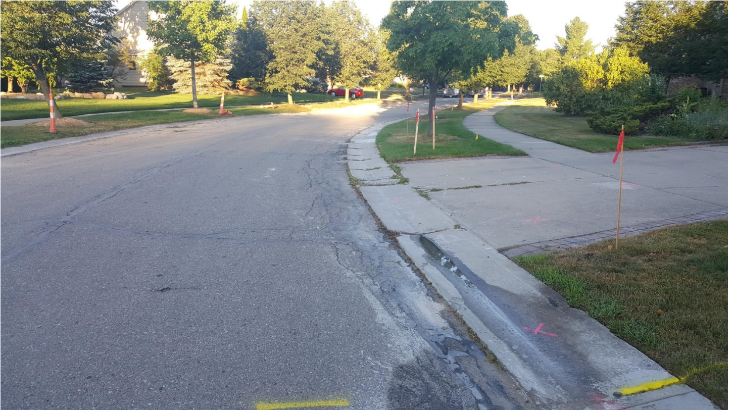
Greenwood Oaks Sub – Nantucket Drive – Pre-Construction
